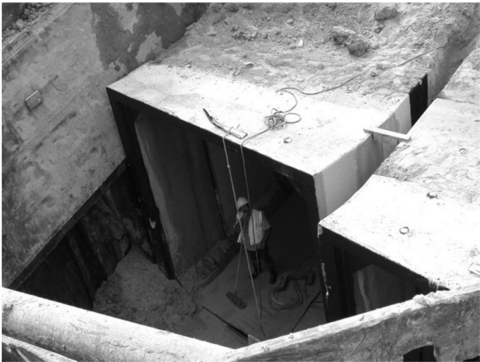
The installation of large new culverts under Kirby, Cambridge, & Hermann
