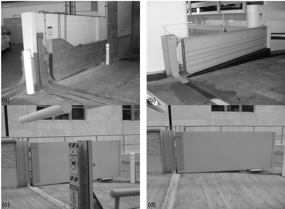
Fig. 7. Recently installed flood gates to keep flood water from getting into some low-lying areas on the TMC campus (images by authors)
