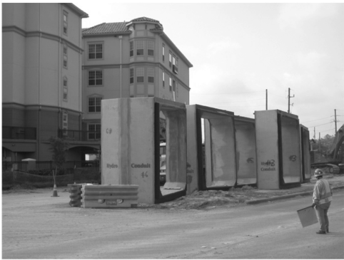
The installation of large new culverts under Kirby, Cambridge, & Hermann
