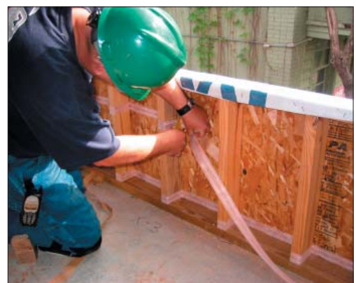
The pair of copper strips on Detec’s moisture detection tape are connected to stainless steel probes so they can sense moisture buildup both on the surface and inside wood framing members. The system can also include temperature sensors to help interpret the moisture data.
