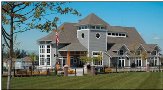
Blakely Hall, which has earned both Green Globes and LEED certification, features low-flow toilets and fixtures, waterless urinals, locally sourced materials, recycled-content materials, and extensive daylighting, among other green features.
