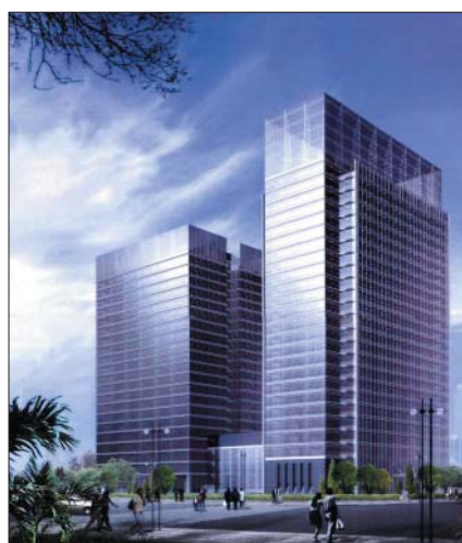
Beijing's Century Prosper Center was the first project to achieve pre-certification through the LEED-CS Rating System. A high-performance chiller, heat-recovery ventilation, and low-emissivity glazing will reduce energy use, and graywater reuse, dual-flush toilets, and waterfree urinals will reduce potable water use. Rendering: RTKL Associates, Inc.
