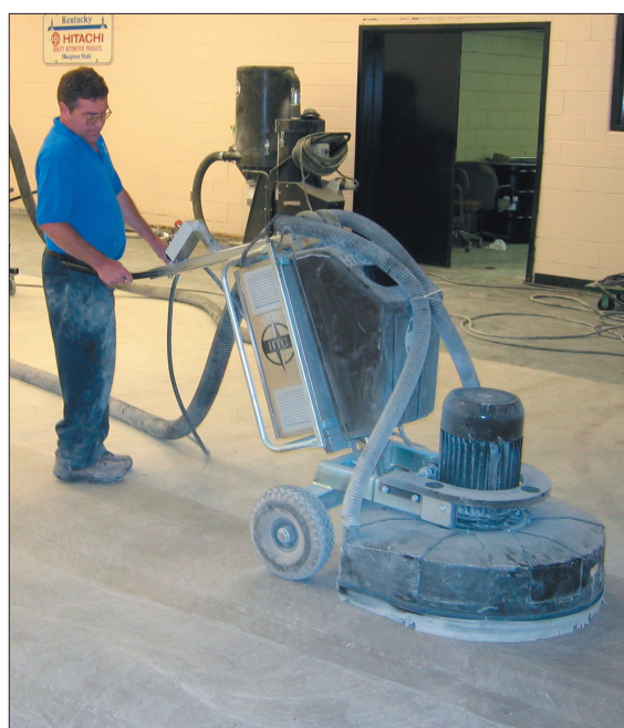
Concrete grinding and polishing relies on highly advanced machines that HTC pioneered in Europe in the early 1990s.
