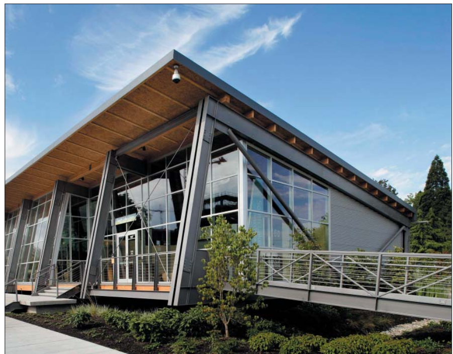
The Pavilion in the Park, located in Seattle, is an exhibition space designed to come apart in modules and move throughout the region as needed.
