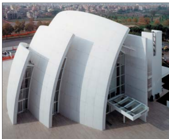
The Jubilee Church in Rome uses TX Active precast concrete panels, which integrate titanium dioxide for a bright white, self-cleaning surface.
