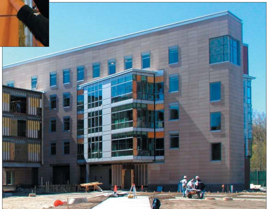
TerraClad is a hollow, fired-terra cotta exterior rainscreen panel for commercial buildings that is installed on an aluminum mounting system.
