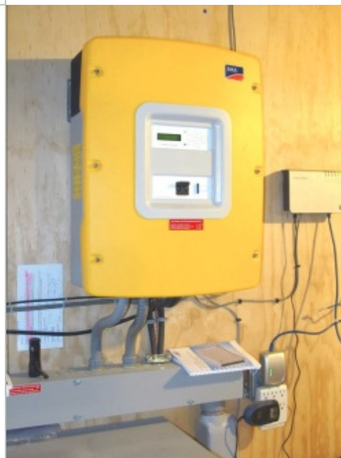
This Sunny Island inverter from SMA America, coupled with a 48-volt battery bank as small as 100 amp-hours, allows a grid-connected PV system to function when the grid is down.
