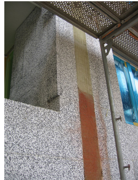
In this assembly, mineral wool is being used as a firebreak between blocks of polystyrene.
