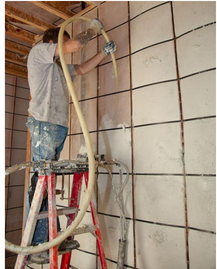
Air Krete is installed in cavities, typically behind webbing, as shown here.
