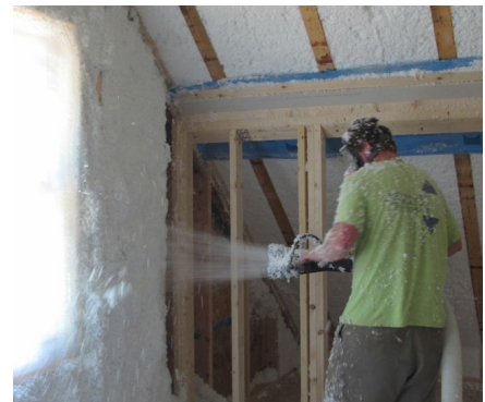
Spider insulation being sprayed into an open wall cavity
