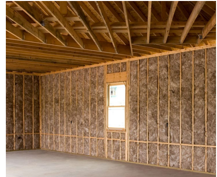
EcoBatt is produced without any dyes, giving the fiberglass a mottled brown appearance.
