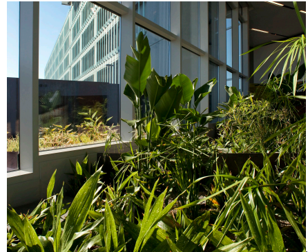
This Living Machine at the ZGF-designed Port of Portland headquarters treats all the wastewater for the building.
