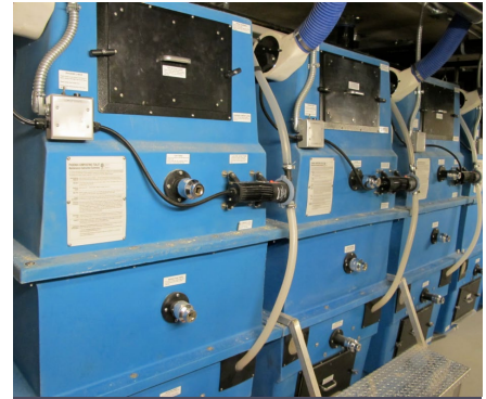
Composting toilets at the Bullitt Center drop waste into these basement composters. Both leachate and compost are taken monthly to amend soil in a nearby forest.
