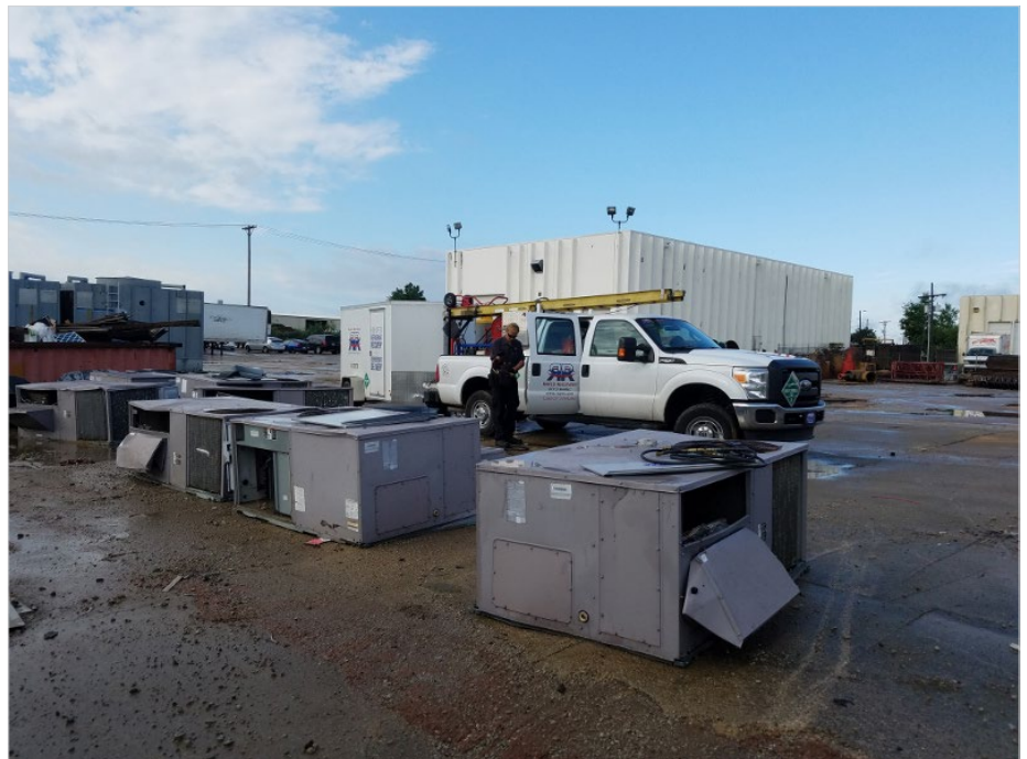
Refrigerant recovery from HVAC equipment.
